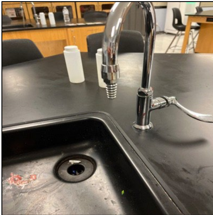
View of potential DWO and sample 04-01-105-CF-P-15 (No sample taken. Outlet was offline.)
