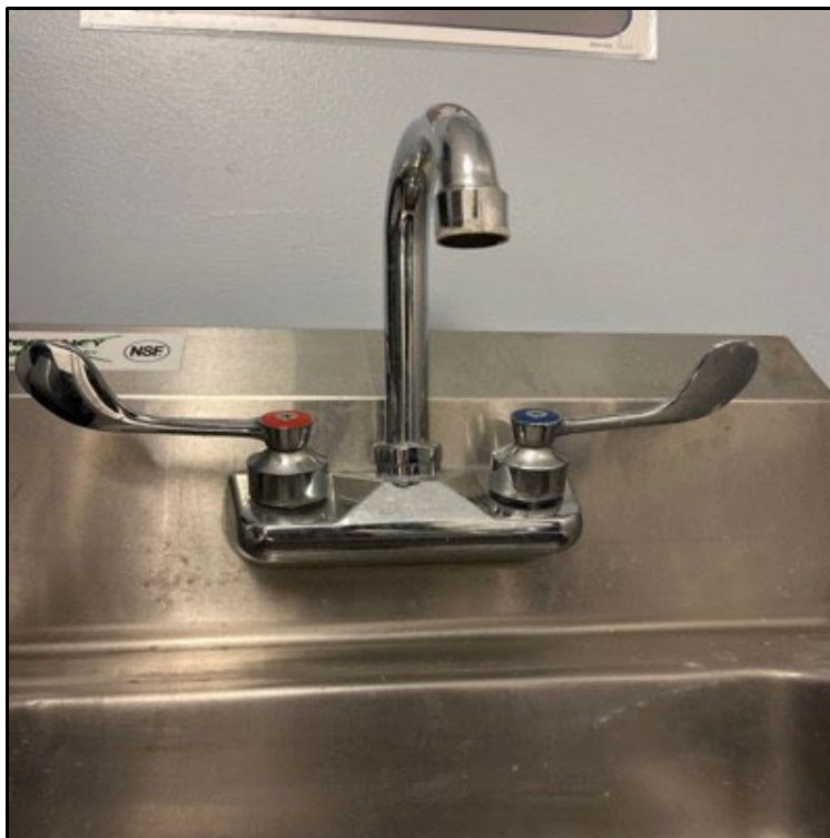
View of potential DWO and sample 04-01-108-HW-P-5
