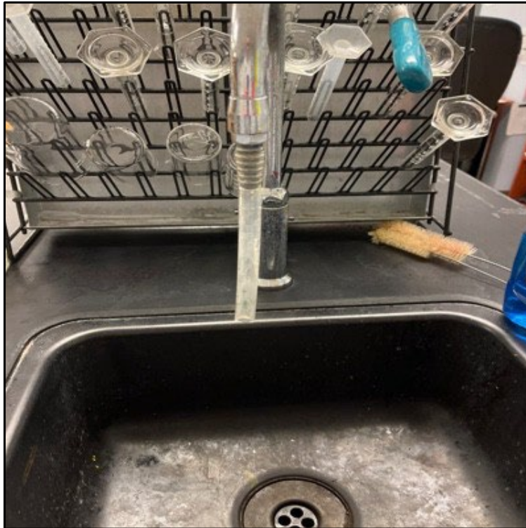
View of potential DWO and sample 04-01-105-CF-P-13 (No sample taken. Outlet was offline.)
